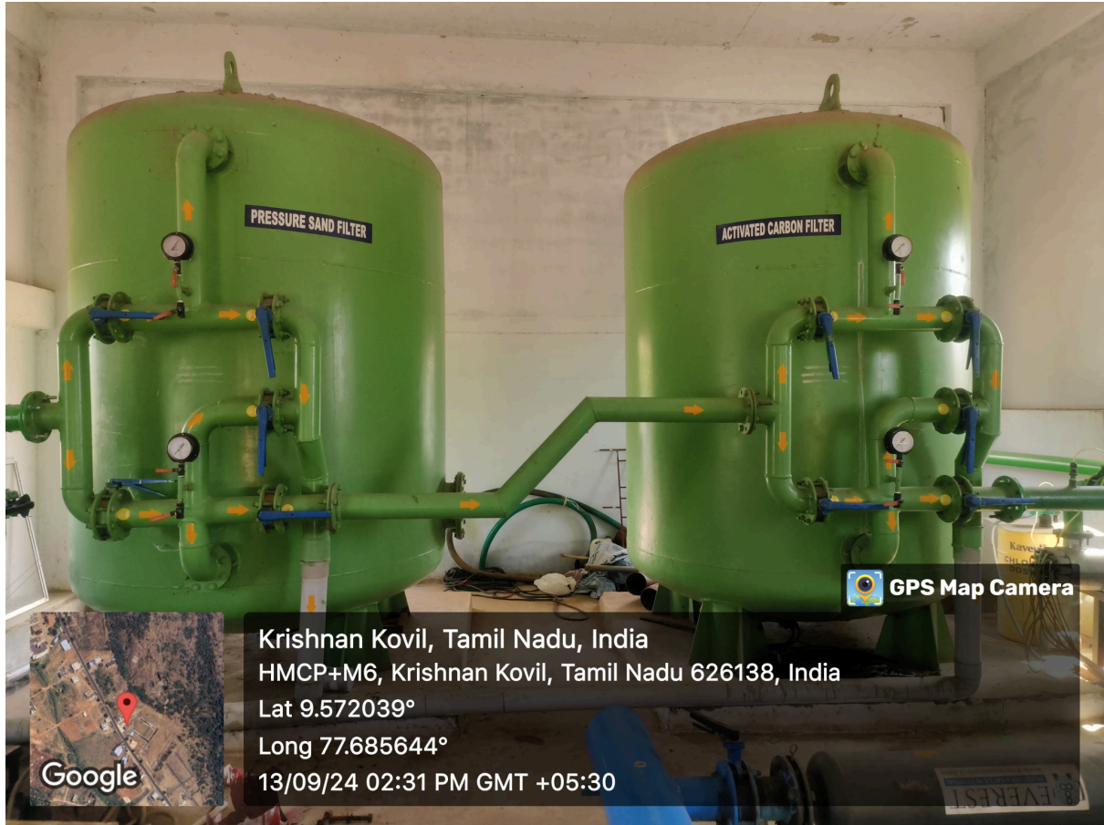
Adsorption Column (Rapid Sand Filter and Activated Charcoal Filter) Facility in the STP at Kalasalingam Academy of Research and Education.
