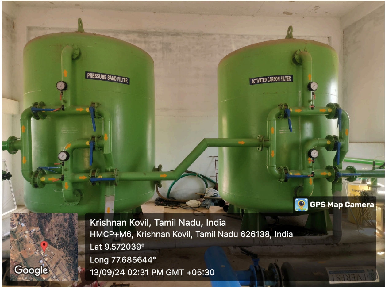
Adsorption Column (Rapid Sand Filter and Activated Charcoal Filter) Facility in the STP at Kalasalingam Academy of Research and Education, TN
