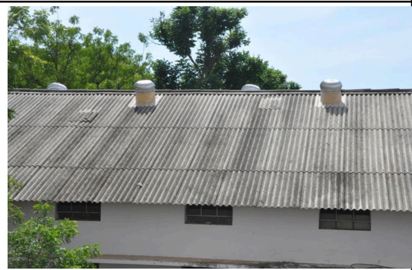
Passive cooling systems using roasting building exhausters.
