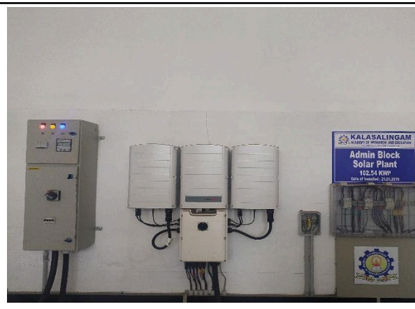
Automatic Solar Energy management system for energy supplies and production – Solar power converters.
