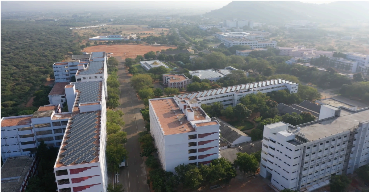
Solar panels in all buildings
