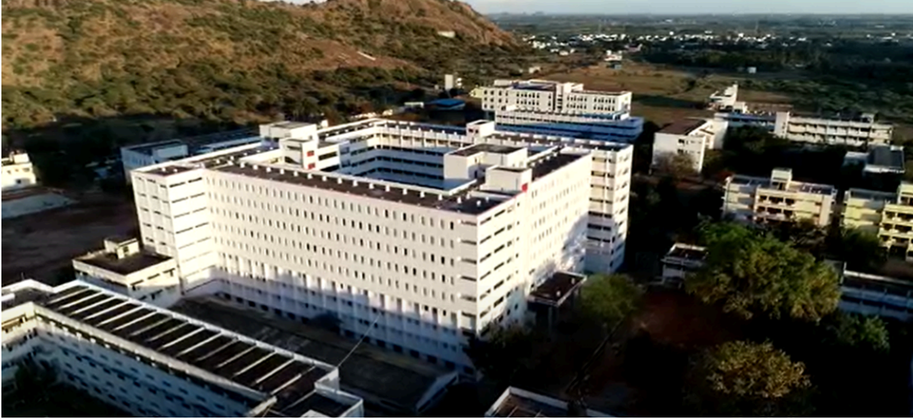
Solar panels in all buildings
