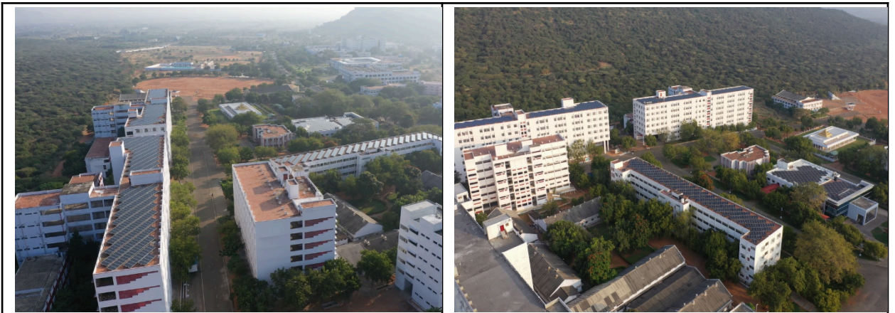
Rooftop Solar plant
