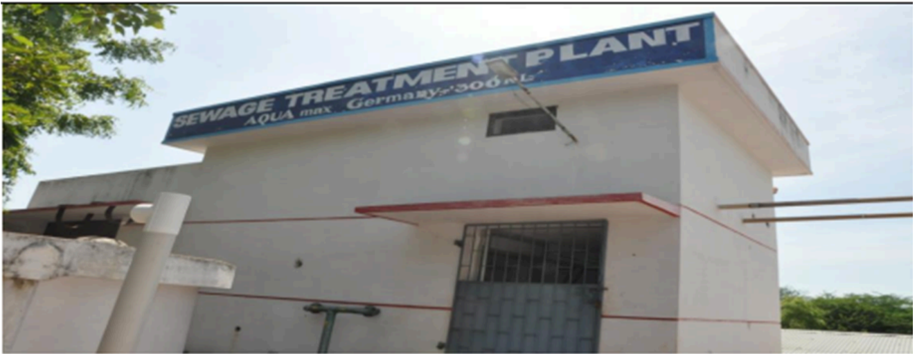
Figure:3 Sewage Treatment Plant 1 – (300 Kiloliter per day)
