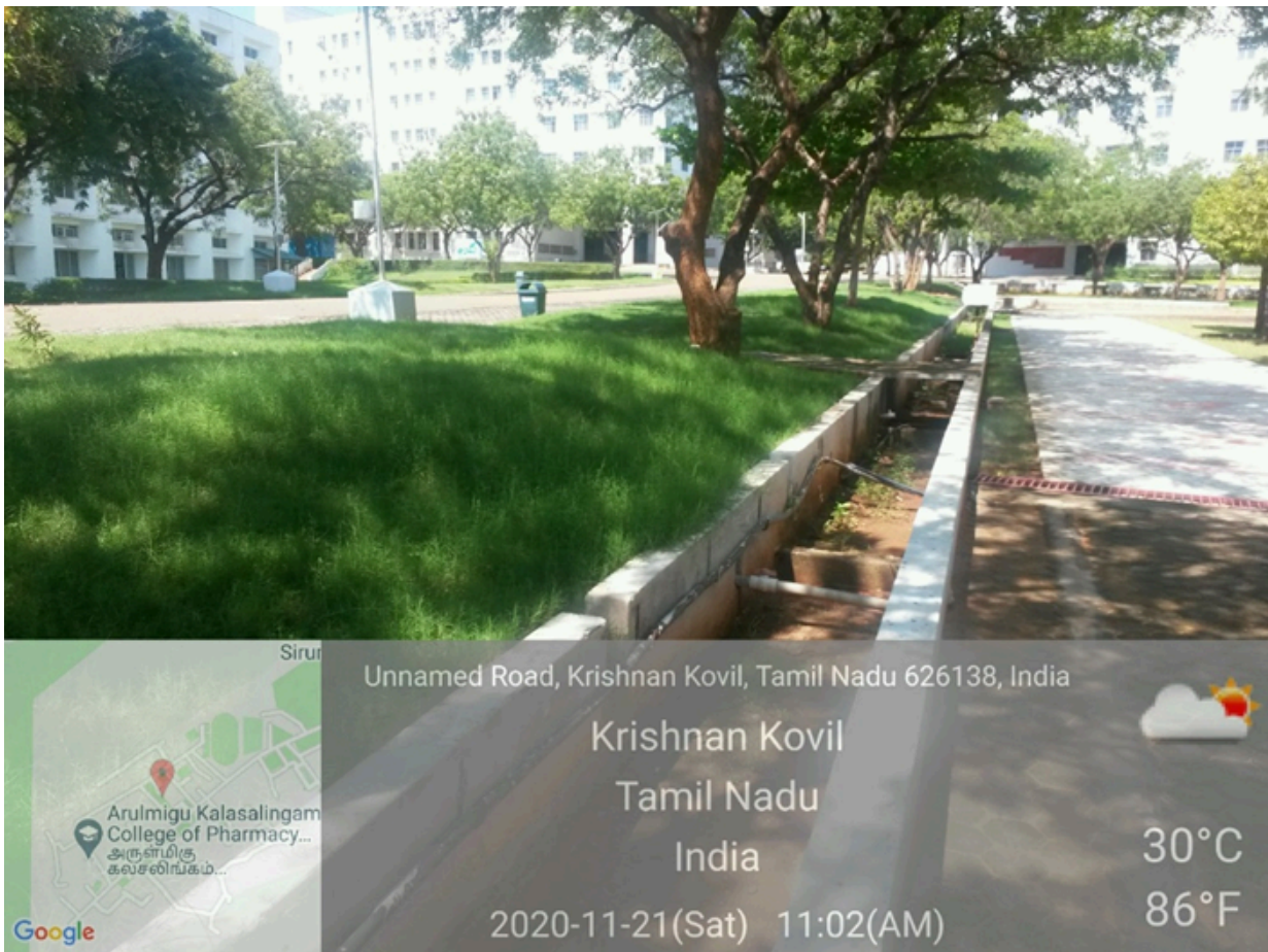
Figure:1 Separate canals for the rainwater collection
