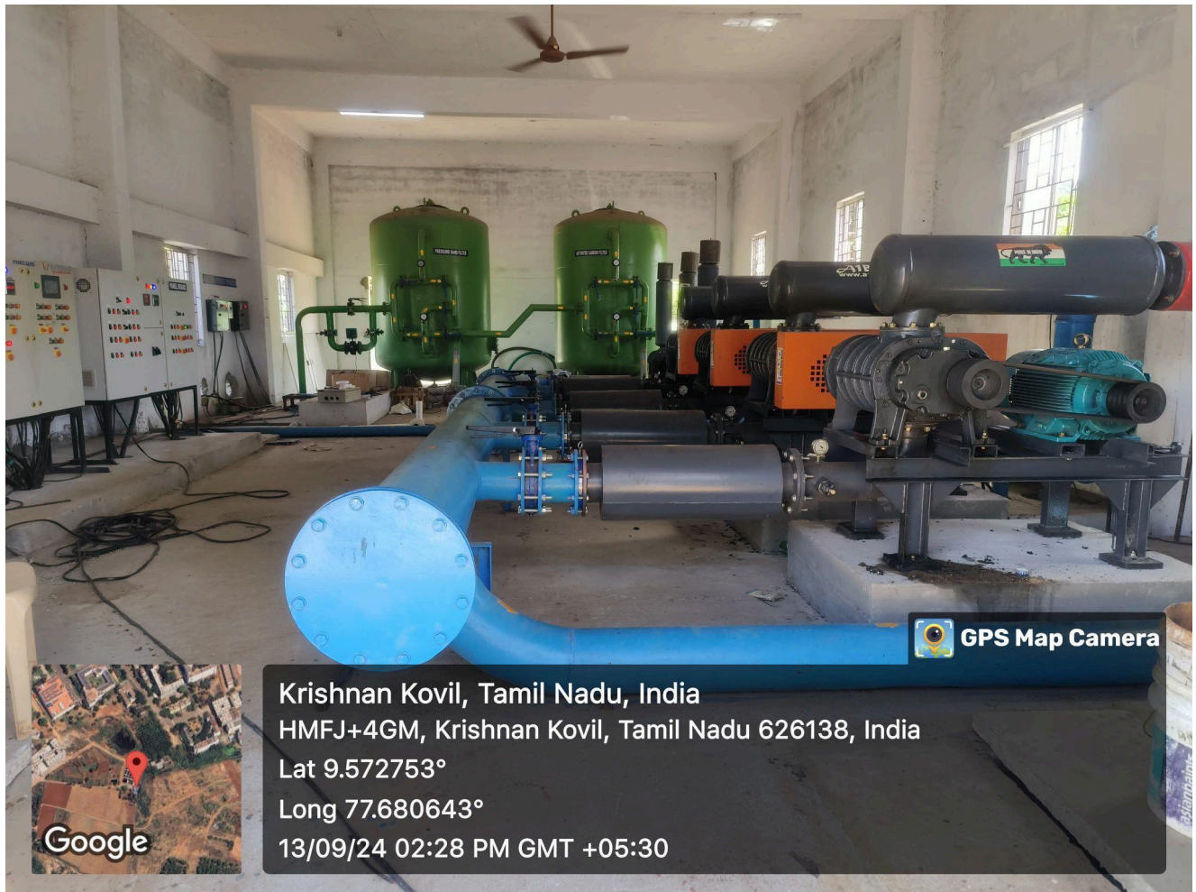
Figure:5 Tertiary treatment of sewage water using rapid sand filter, activated charcoal, UV and Chlorine disinfection
