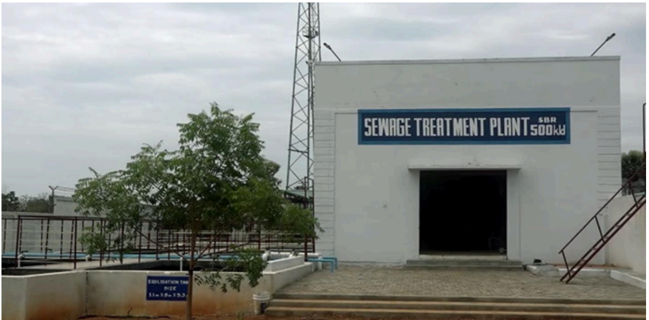
Figure:4 Sewage Treatment Plant 2 – (500 Kiloliter per day)
