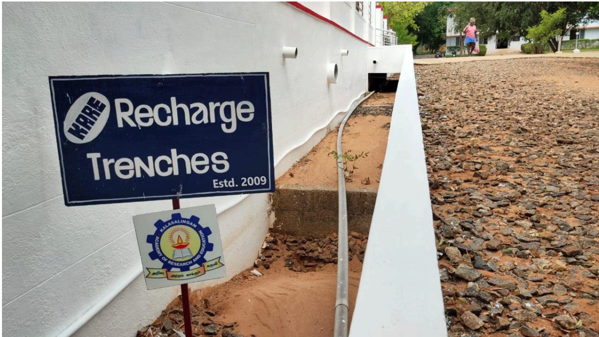
Recharge Trenches near Manimandapam
