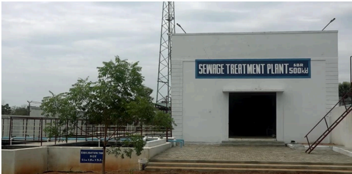
Sewage Treatment Plant – (500 Kiloliter per day)
