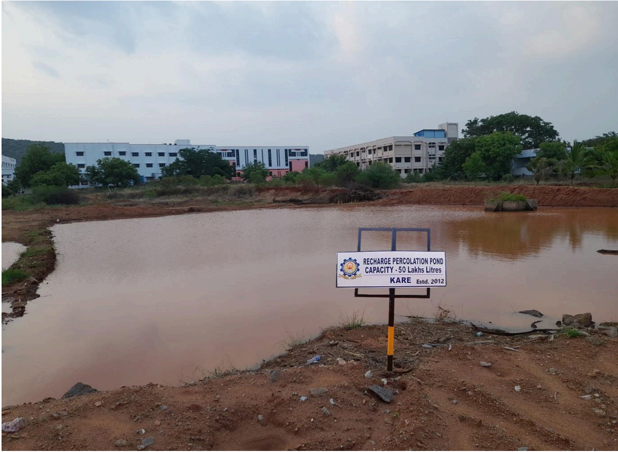
Recharging Percolation Ponds Location at Babbage Block / Academic Block-VI
