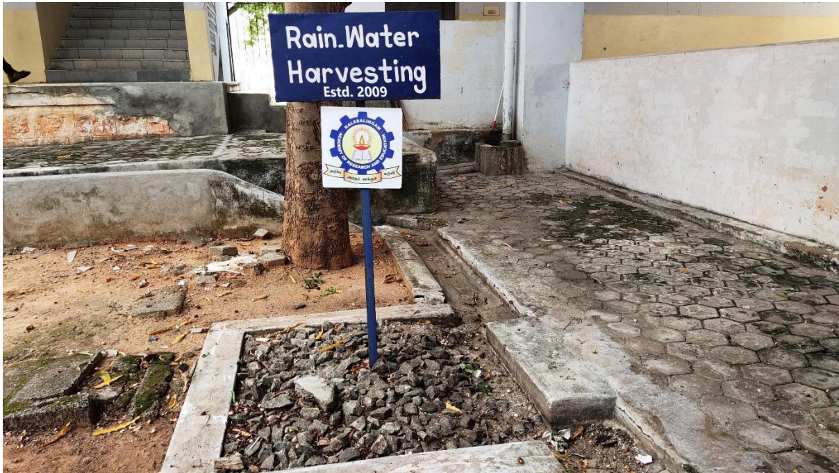
Rainwater Harvesting System near Srinivasa Ramanujan Block / Academic Block-VIII
