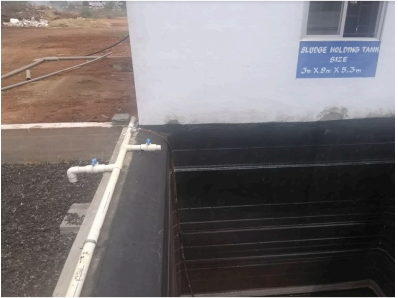
Figure 7: Sludge Digestion and Sludge Drying Bed
