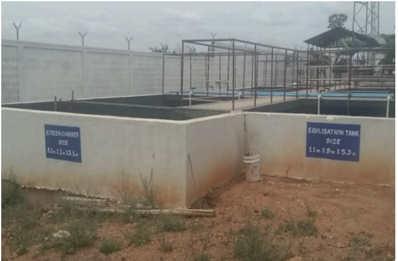
Figure 4: Equalization Tank (5 KLD)
