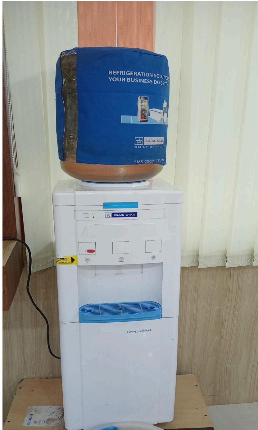
Water cooler/Heater available in each blocks
