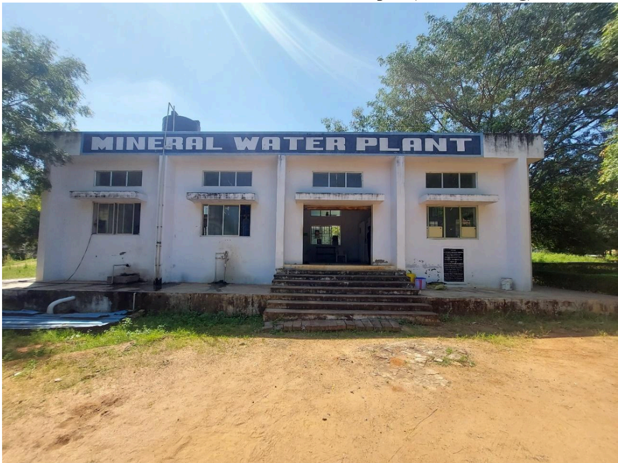
Mineral Water Plant at KARE Campus (Old Building)
