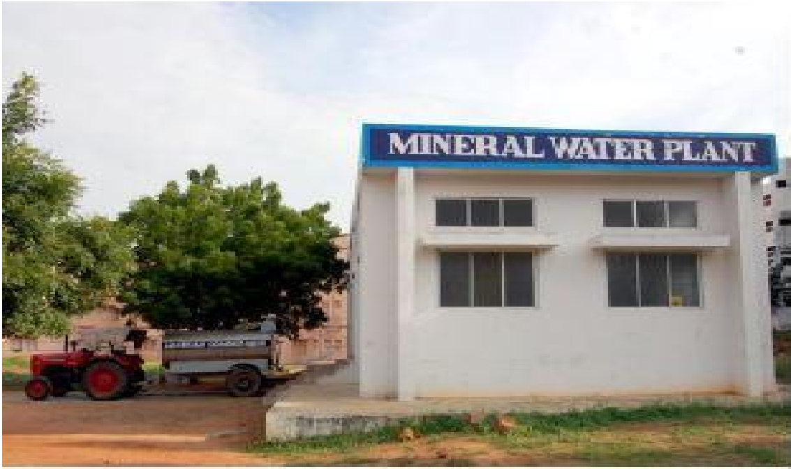
Mineral Water Plant at KARE Campus (New Building)
