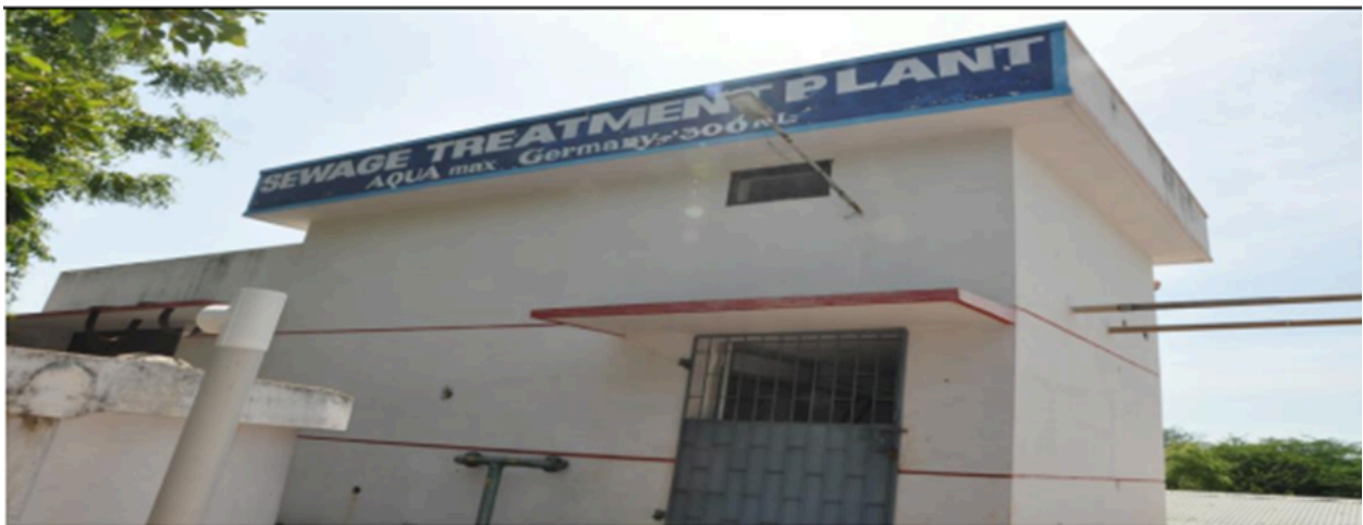
Sewage Treatment Plant 1 – (300 Kiloliter per day)
