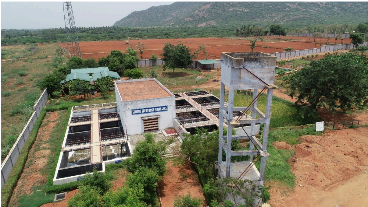
Overview of Sewage Treatment Plant
