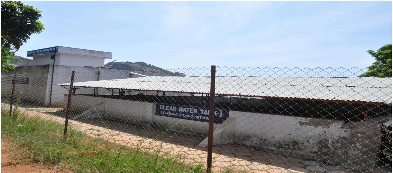
Waste Water Treatment and Clear water Storage facility in Kalasalingam Academy of Research and Education
