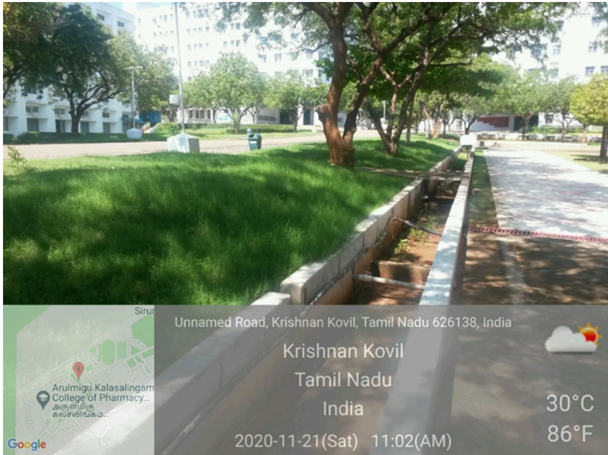
Figure:1 Separate canals for the Rainwater collection and Transportation
