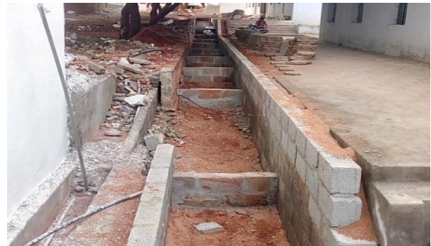
Construction of rainwater harvesting facility
